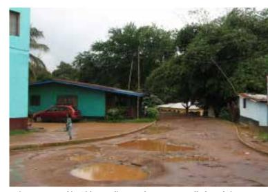
Figure 74. Road in Old Matadi. Note that even metalled roads in government-developed housing areas have little drainage, in one of the wettest countries in the world
