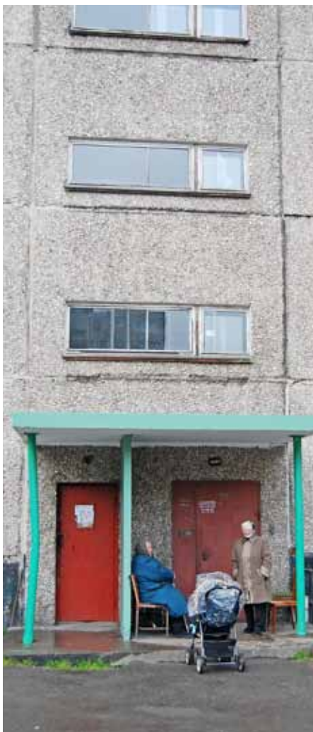
A large part of the housing stock in central and eastern Europe are panel houses, built from low-quality materials and in great need for renovation.
