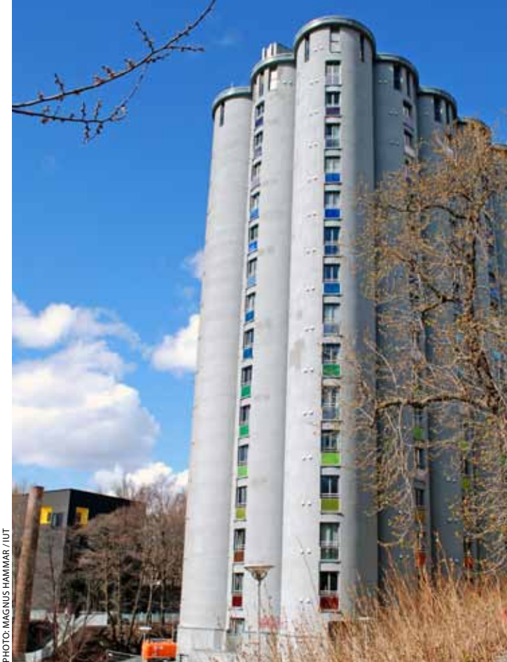
This grain-silo from 1954, in the area of Grünerløkka in Oslo, was rebuilt in 2001 to be made habitable. It now serves as a dormitory for students. New floors were made, holes for windows were cut and custom furniture were made to fit correctly in 229 flats.
