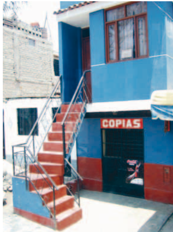
Rental unit combined with commercial unit, self built in a popular neighbourhood in Lima, Peru. Photo © UN-HABITAT/ Claudio Acioly Jr.
