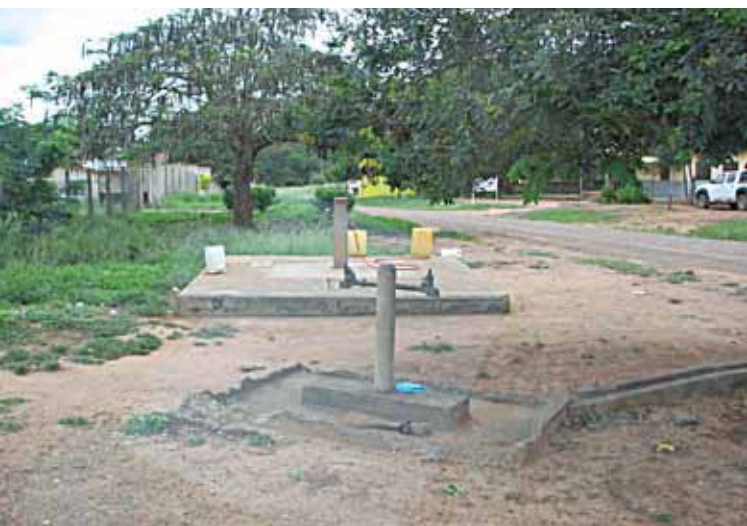
Figure 37. Public standpipe on the outskirts of Accra.
