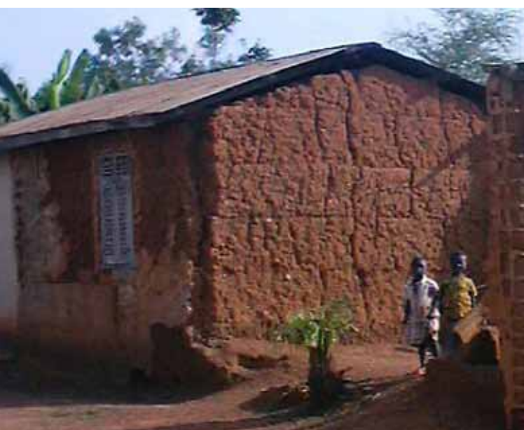
Figure 55. Laterite built as atakpamé Photo © Royal Danish Academy of Fine Art
