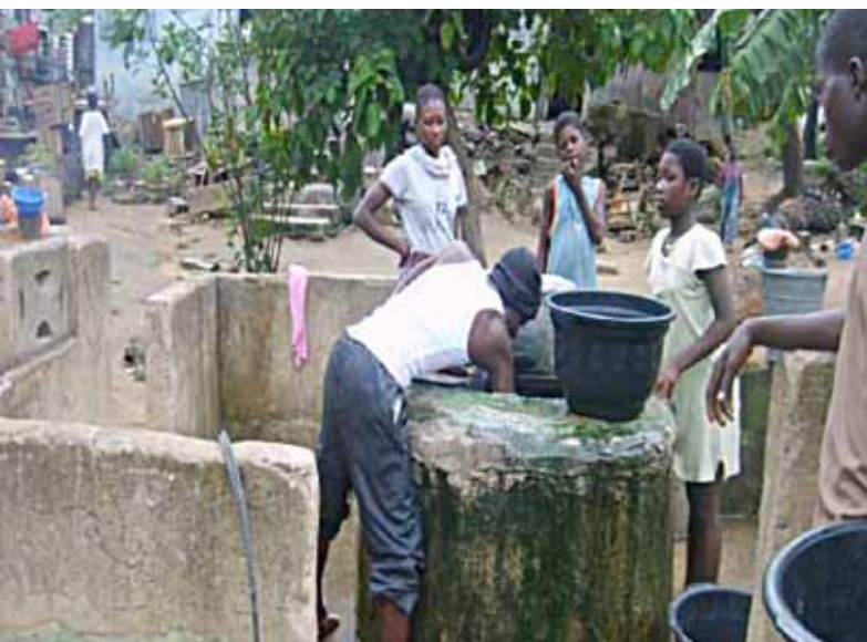
Figure 38. A shallow hand dug well in Dome, Accra. Photo © M. Oteng-Ababio
