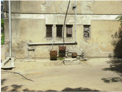
3 Individual water pumps to boost supplies to upper floors. Note the paint peel offs and obstructed toilet windows to the ground level unit
