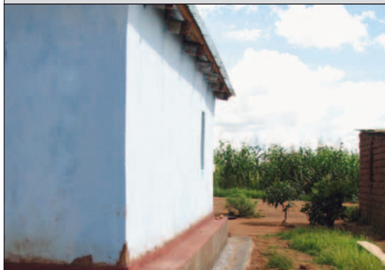
Figure 47. Good quality adobe walling, well plastered, high quality foundations and drainage and adequate roof overhand. CCODE Area 49, Lilongwe
