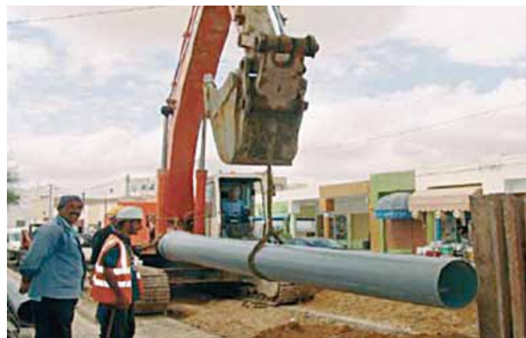
Figure 8.4 Installation of collector sewers
