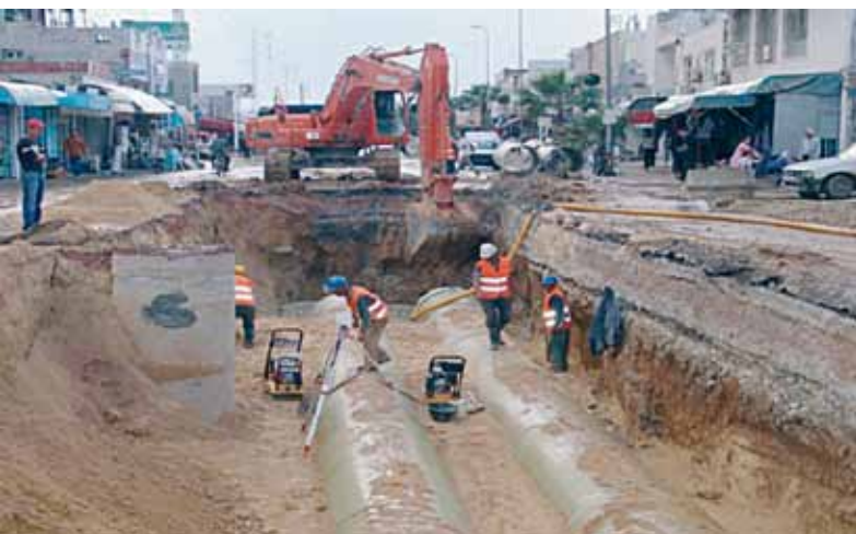
Figure 8.3 New sewerage main under construction
