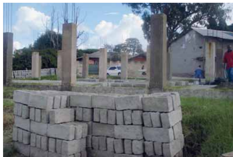
Figure 75. Informal construction with blocks and in situ concrete columns, Kitwe. Photo © UN-Habitat/Daniel Phiri
