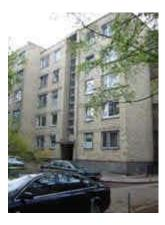
Construction principles: Brick walls, flat roof, wooden windows with double glasses Heat supply: Heat substation with hot water preparation in the building
