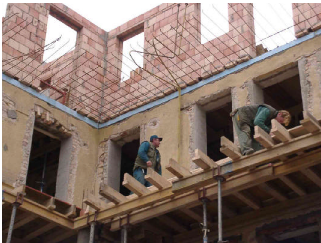
Renovation of an old building in Budapest, Hungary. The building has been re-used and adapted by adding an extra floor (uptopping).
