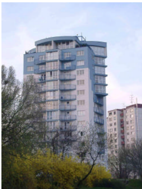
Old (right) and renovated (left) apartment blocks in Bratislava, Slovakia
