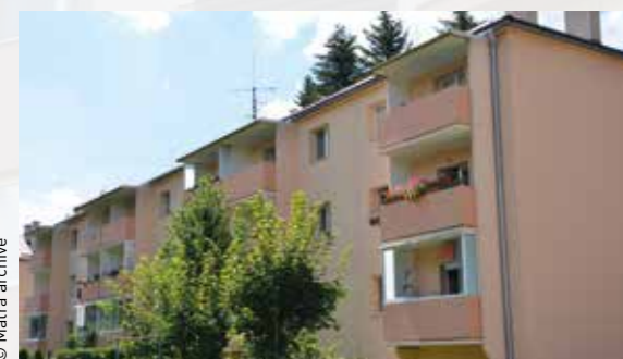
Renovated and modernised building
